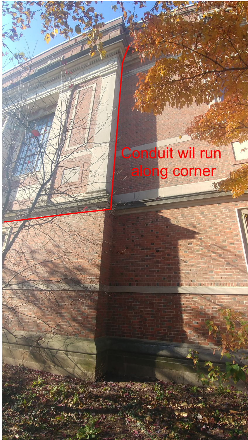
Conduit run along building to AP
