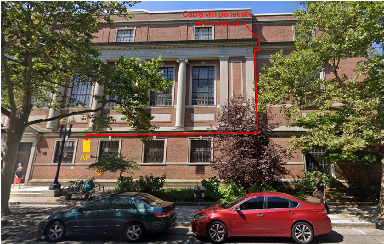
Cable run from 3 rd Floor “Cube Rm” CEN switch to AP
